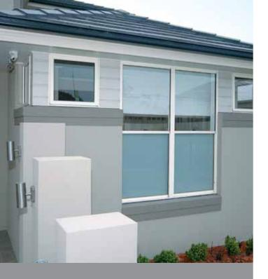
With an adjustable top and bottom hung sash, Stateman's **double hung window** provides superior climate control performance, allowing you to direct air through the top, bottom, or both sashes together.
